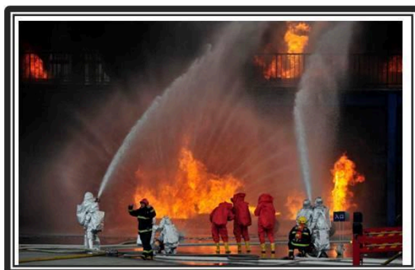
Picture showing front side of the factory on fire
